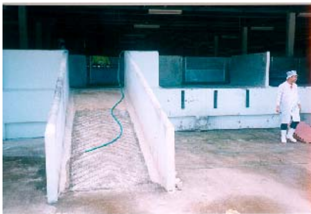
Fig. 16: Ramp for pigs and off-loading platform for vehicles leading to holding pens for pigs
