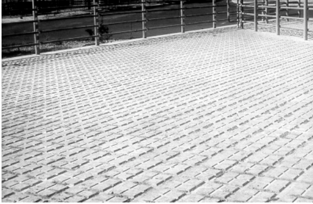
Fig. 23: Non slip concrete pen floor partition
