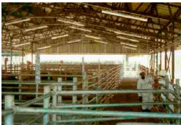
Fig. 21: Smooth tubular rails for pen partitions
