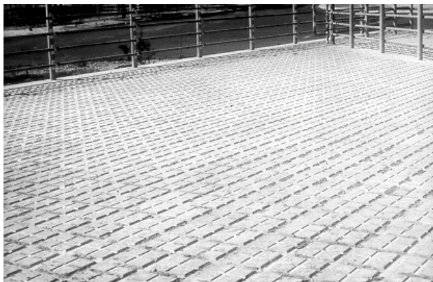
Fig. 23: Non slip concrete pen floor partition
