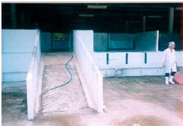
Fig. 16: Ramp for pigs and off-loading platform for vehicles leading to holding pens for pigs
