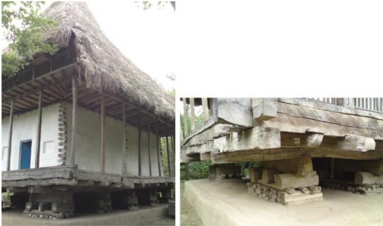
Fig: 3 Sliding Isolator
