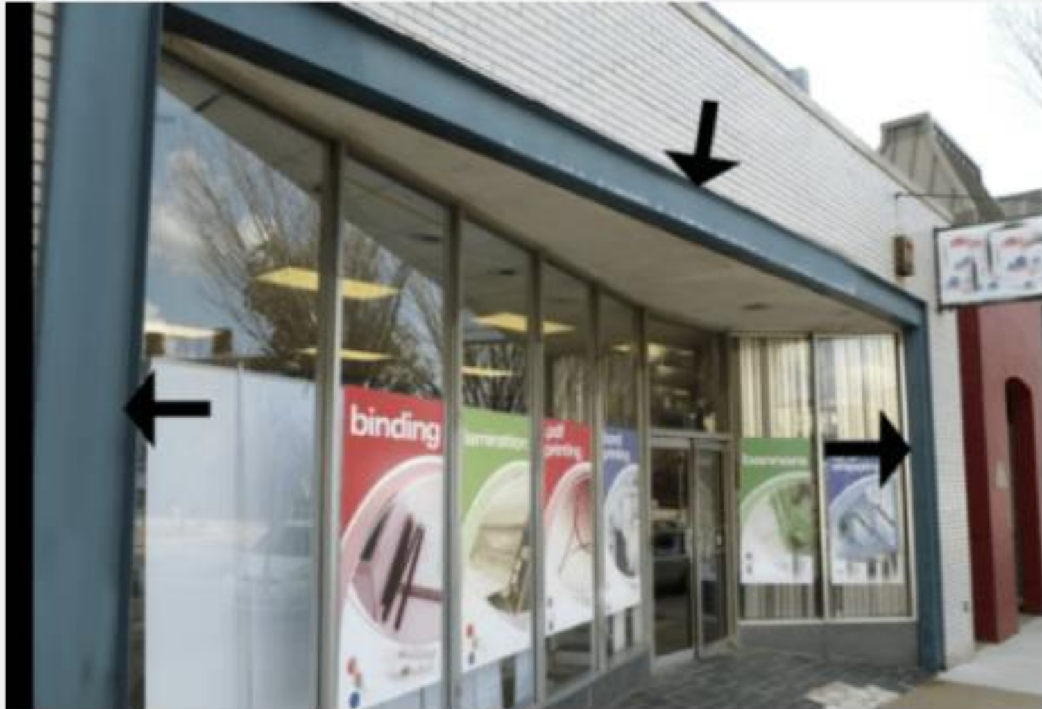
Large building entryway moment frame
