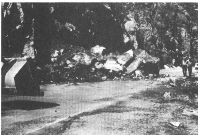
Figure 8b. Rockfall on U.S. Highway 6, Colorado (photograph by Colorado Geological Survey).
