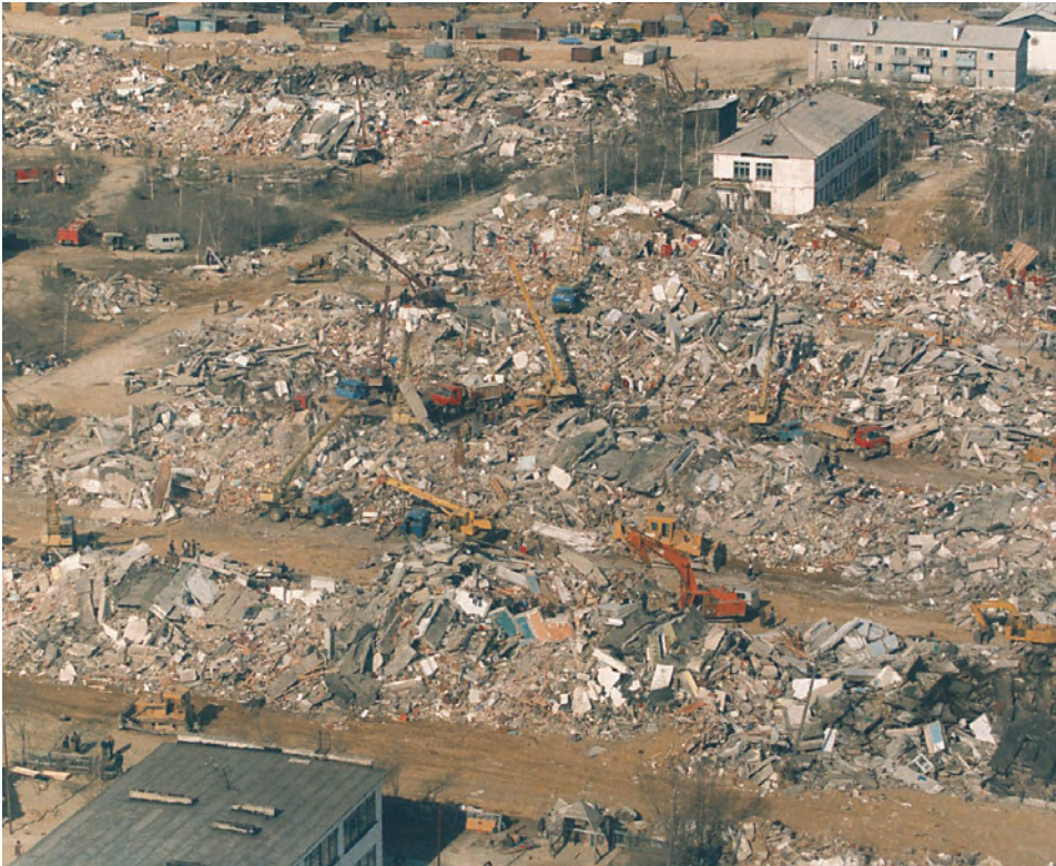
Figure 6.22 Buildings collapse in Russia Rows of prefabricated, unreinforced, five-story apartment buildings destroyed by the 1995 earthquake that struck the island of Sakhalin in Russia (M 7.5). (Tanya Makeyeva/AP/Wide World Photos)
