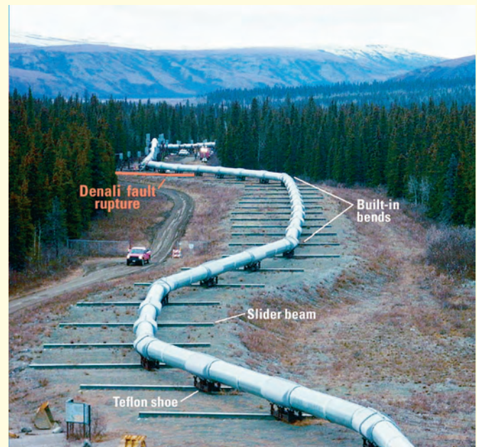
Figure 6.E A Trans-Alaska oil pipeline survives (M 7.9) earthquake The Alaskan pipeline was designed to withstand several meters of horizontal displacement on the Denali fault. The 2002 earthquake caused a rupture of 4.3 m (14 ft) beneath the pipeline. The built-in bends on slider beams with teflon shoes accommodated the rupture as designed. This was strong confirmation of the value of estimating potential ground rupture and taking action to remove the potential threat and damage. [Alyeska Pipeline Service Company (ASPC)]
