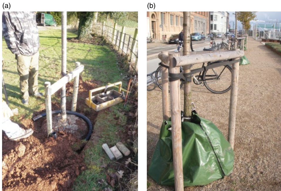
Figure 6.2 (a) An irrigation tube being installed in a tree planting pit. (b) A watering bag placed around a recently planted tree in Copenhagen, Denmark. The bag has a porous base that slowly releases water to the root ball and surrounding soil over a number of hours. This helps reduce surface run-off and ensures deeper soil water recharge. Here, a Tregator® bag is being used, but a number of different brands and designs are available.
