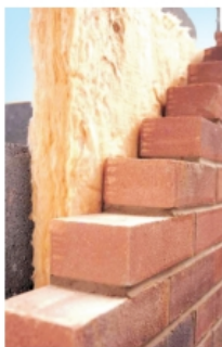
Figure 9.5: Soft insulation board between external brick wall of a house.
