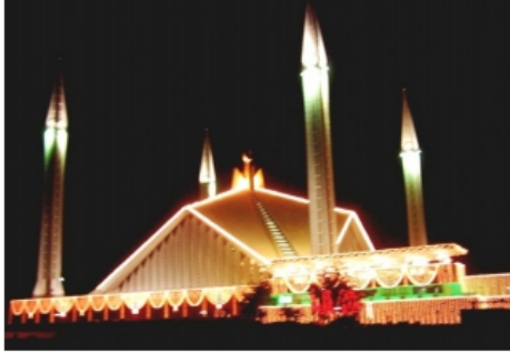
Figure 6.11: Light is needed during night also.
