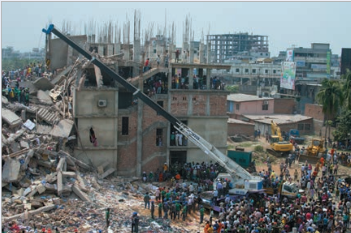
Shirts with the Benetton label were found in the rubble of a collapsed Bangladesh garment factory.
