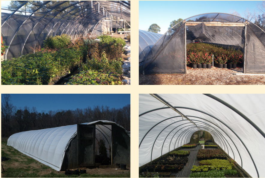
Figure 13. (top) Plants in a coastal plain ecoregion are pushed together beneath a structure covered with shade cloth. (bottom) An overwintering structure 22' wide by 96' long is covered with one layer of 4 mil white polyethylene. The ends are made of wood, and ventilation is created by opening the doors at either end of the house.
