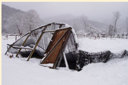
Figure 17. Winter protection houses collapsed by snow load. The greenhouse in the left-hand photograph and the greenhouse on the right side of the right-hand photograph were covered with shade cloth, which accumulates snow load more quickly than plastic. In this particular heavy snow accumulation, the house covered with plastic on the left side of the right-hand picture also collapsed, although not as severely. These collapses occurred within hours of snow beginning to fall.
