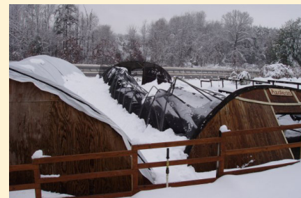
Figure 17. Winter protection houses collapsed by snow load. The greenhouse in the left-hand photograph and the greenhouse on the right side of the right-hand photograph were covered with shade cloth, which accumulates snow load more quickly than plastic. In this particular heavy snow accumulation, the house covered with plastic on the left side of the right-hand picture also collapsed, although not as severely. These collapses occurred within hours of snow beginning to fall.
