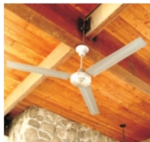
Figure 4.32: A ceiling fan rotating at constant speed is in equilibrium as net torque acting on it is zero.
