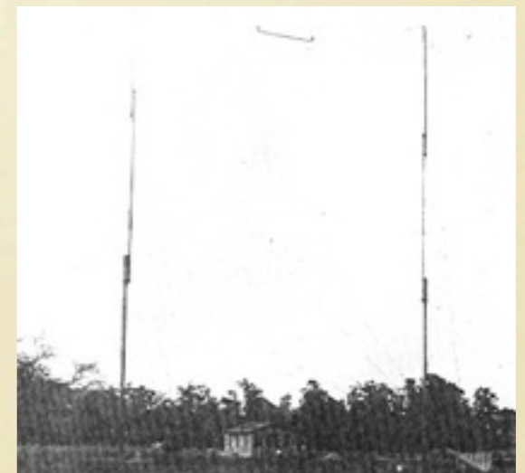
Twin radio towers at Cobb Island
