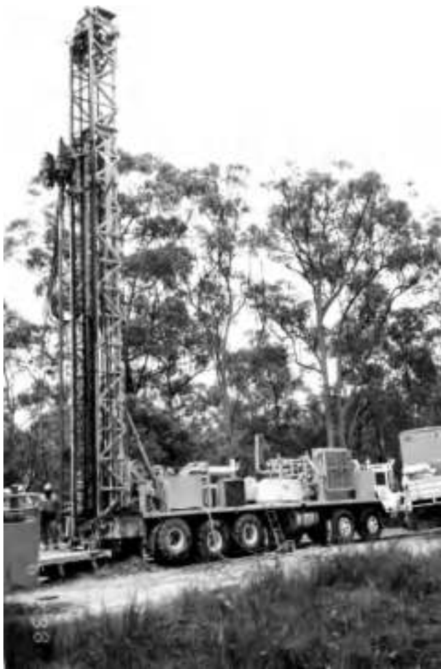
Figure 6.24 Truck-mounted drill rig, here employed in coal exploration in the Sydney basin, New South Wales, Australia. Courtesy of Keith Bartlett, Minarco-Mineconsult, Tuggerah, NSW.
