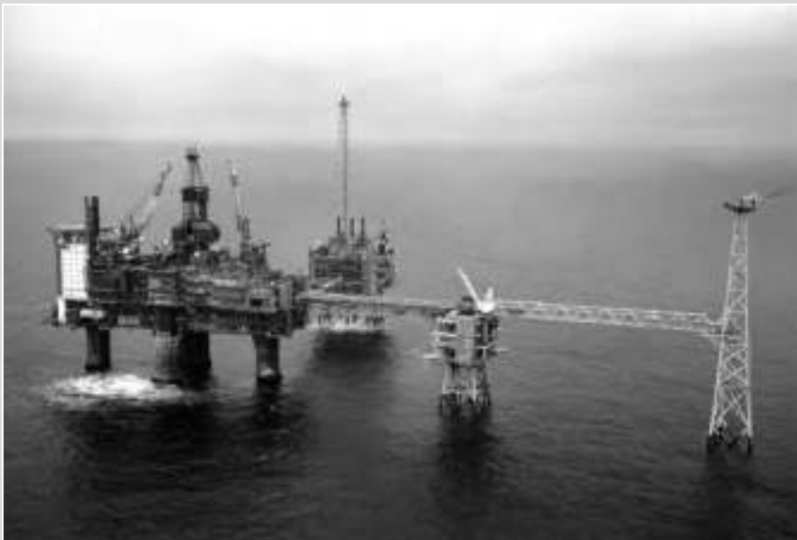
Figure 6.2 (Plate 6.2) Sleipner platform in the North Sea off Norway is the world's first large-scale geological CO 2 sequestration operation. On the platform, carbon dioxide is separated from natural gas and pumped into a sub-seafloor aquifer. © Øyvind Hagen, Statoil.
