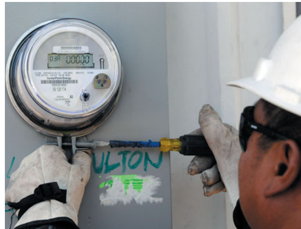
A smart meter being installed
