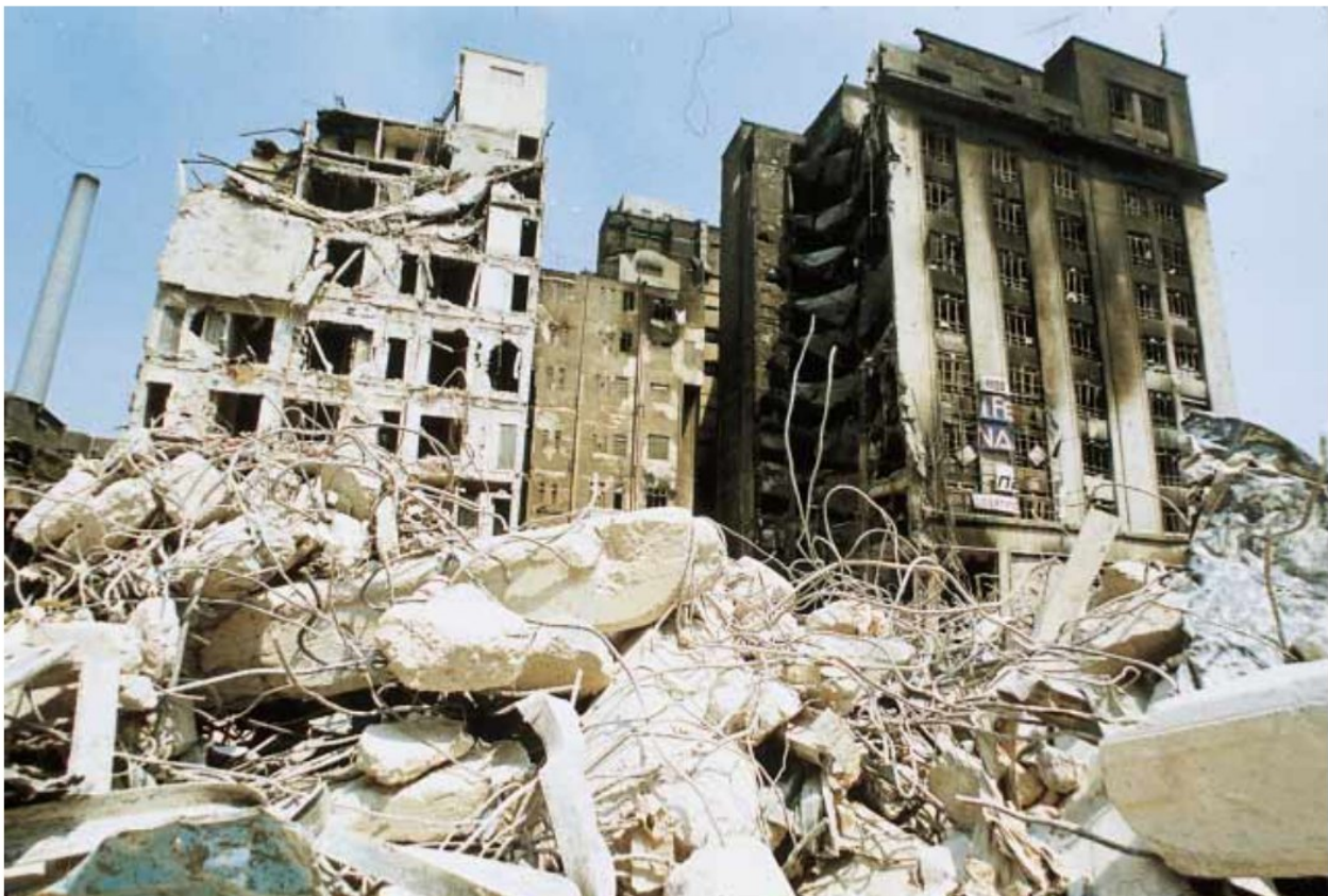
Figure 10–16 The 1985 Mexico City earthquake had a magnitude of 8.1 and killed between 8000 and 10,000 people. Earthquake waves amplified within the soil so that the effects were greater in Mexico City than they were in Acapulco, which was much closer to the epicenter. (AP/Wide World Photos)
