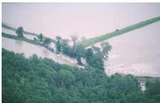
Figure 14–29 Flood waters pouring from the channel of the Missouri River through a broken levee onto the flood plain in Boone County, Missouri. (Stephen Levin)
