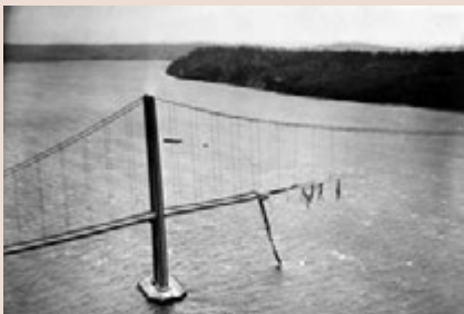
Collapse of the Tacoma Narrows Bridge
