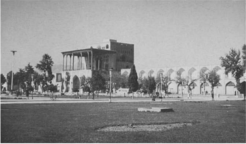
28 (a) Isfahān, the 'Ali Qapu palace, early eleventh/seventeenth century.
