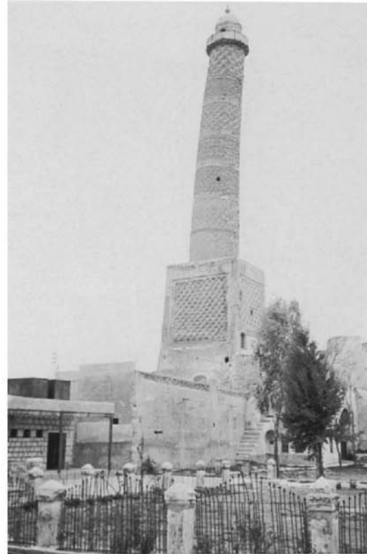
(b) Mosul, the Great Mosque, 543/1148, the minaret.
