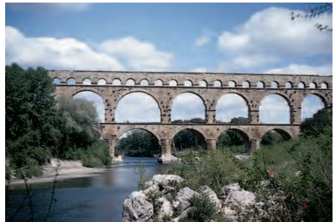
Figure 9.14 Nîmes, France. Aqueducts outside of Nîmes, France were built during the Roman Empire, about 2000 years ago. © Alexander B. Murphy.
