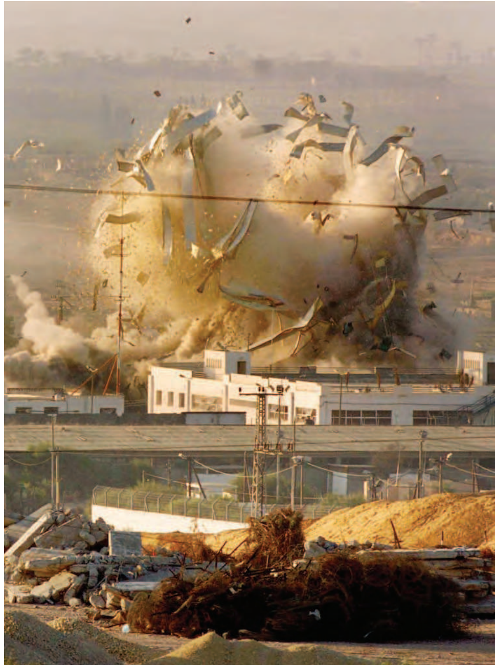
Figure 7.35 Erez Crossing, Gaza Strip. The Israeli Army withdrew from the Gaza Strip in 2005, after occupying the territory for 38 years. Israeli troops demolished the Israeli Army liaison offices on September 9, 2005, in preparation for completing the Israeli retreat from the Gaza Strip on September 11, 2005. © AP/Wide World Photos.
