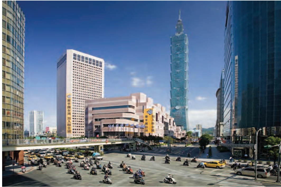
Figure 4.21 Taipei City, Taiwan. The Taipei 101 Building, the World's tallest building. ©José Fuste Raga /Age Fotostock America, Inc.
