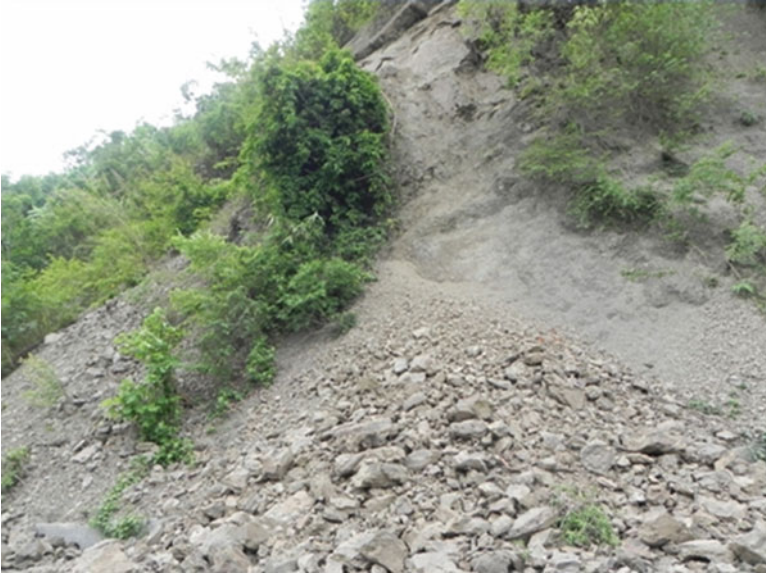
Fig. 3.6 Landslide on a hillslope (Photo courtesy of Dr. Animesh Biswas)
