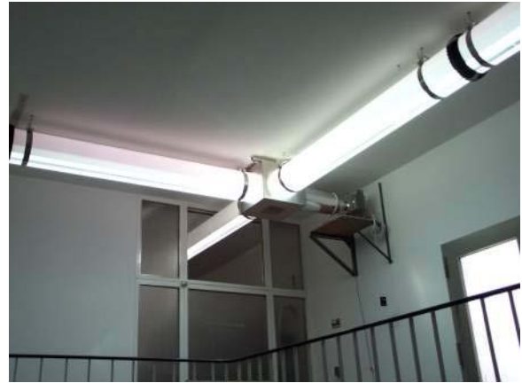
Figure 5-29. Pictures from an Artheliop project installation in Berlin. The heliostat on the roof supplies the light pipe with concentrated sunlight (left). An electrical light source supplies the light pipe with electrical light when needed (right).
