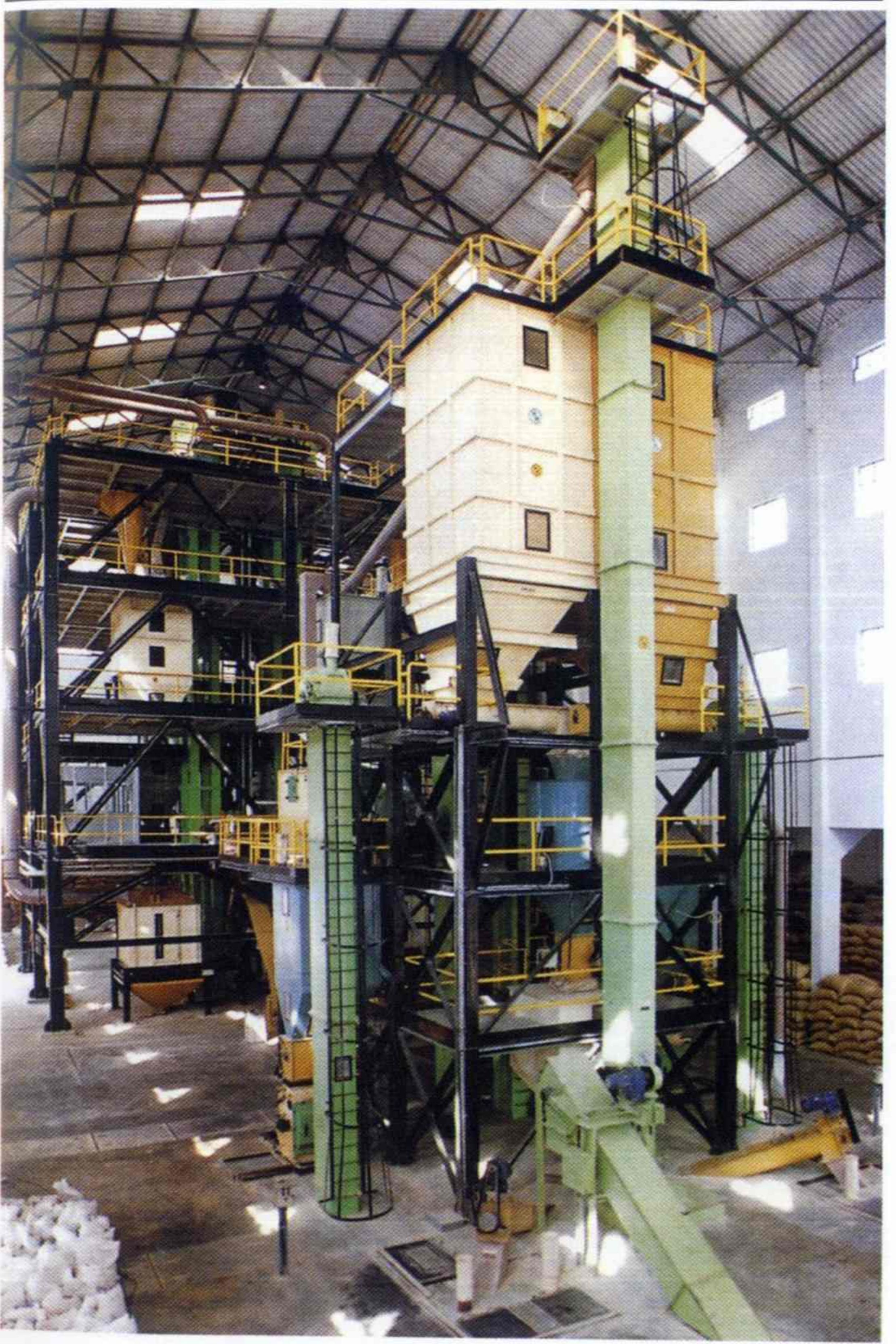
42. Typical large feed mill to produce pellet feed
