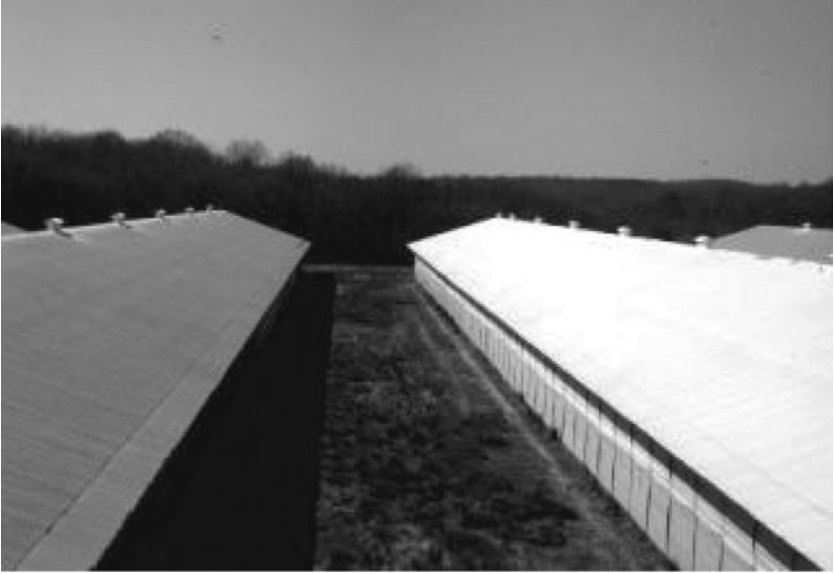
Fig. 5.10. Reflective roof coating.
