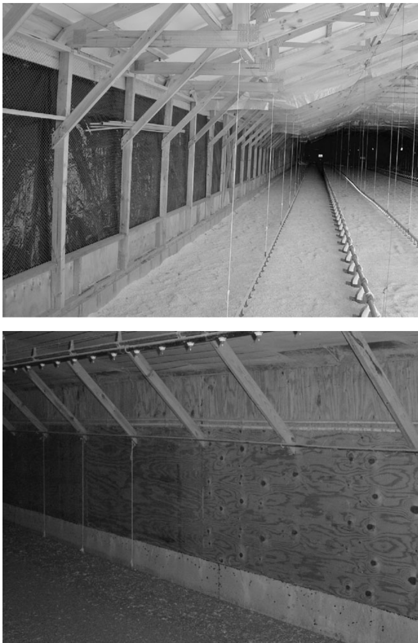
Fig. 5.22. Examples of 'rough' and 'smooth' side walls.
