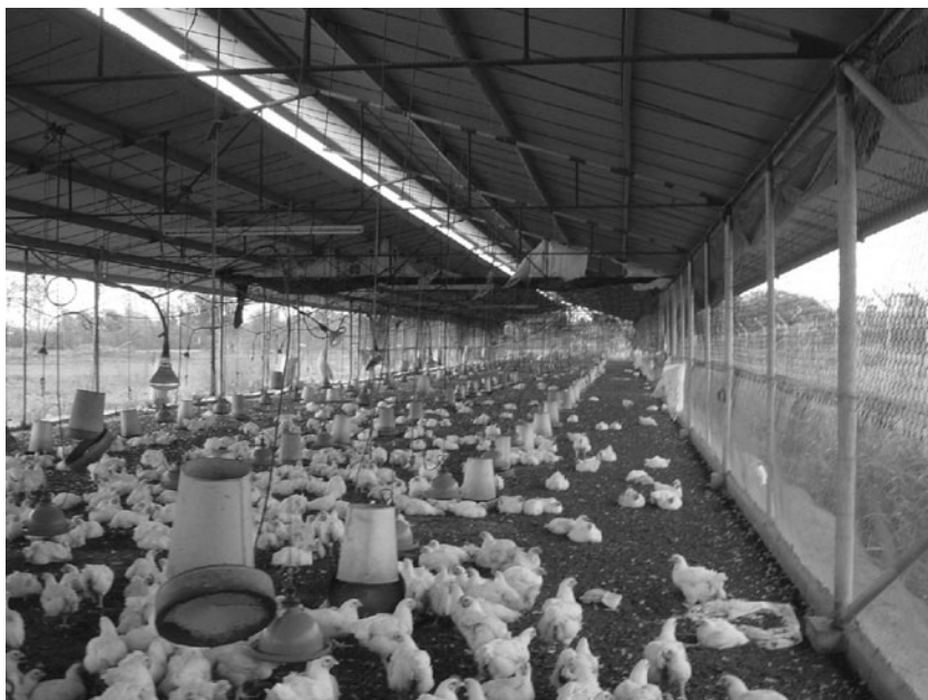
Fig. 5.6. Ridge vent in uninsulated poultry house.
