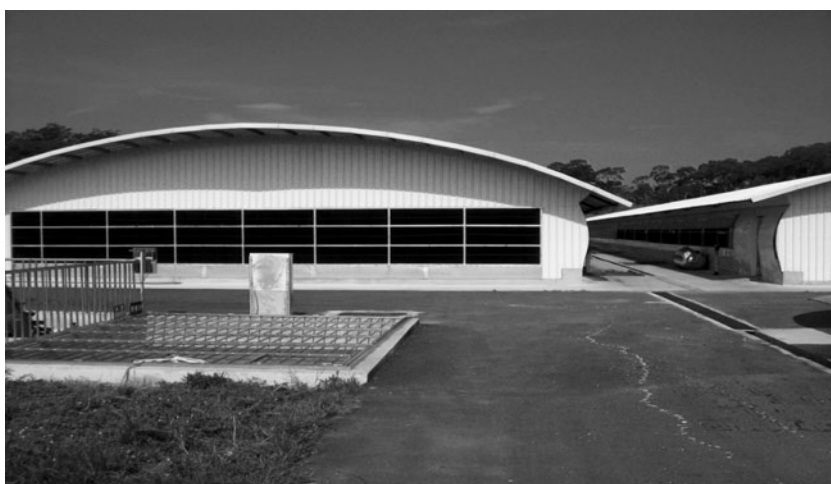
Fig. 12.5. A water-pad cooling/tunnel air system.
