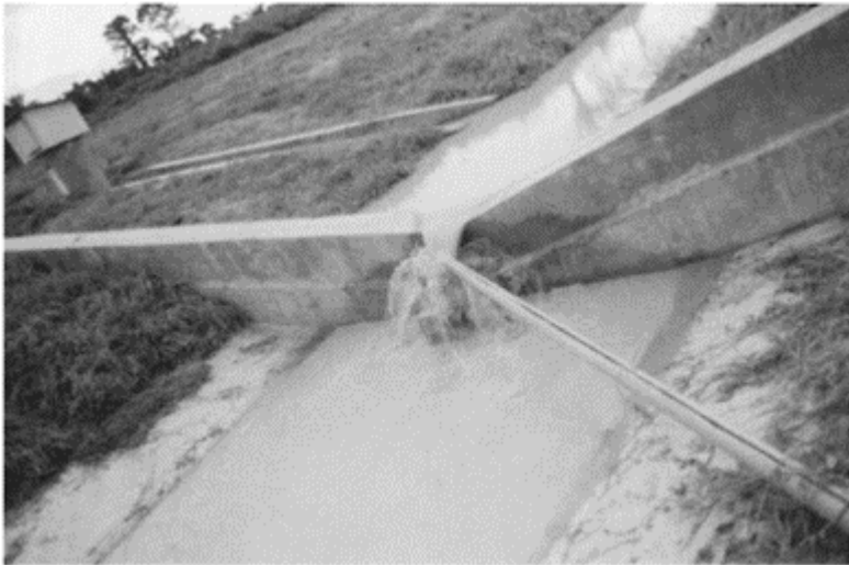
FIGURE 9.17 A weir with a slot-pipe to collect runoff sample.
