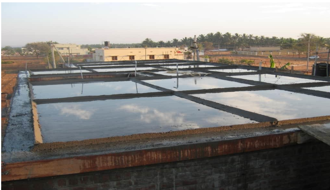
Fig 08: Curing by Pond
