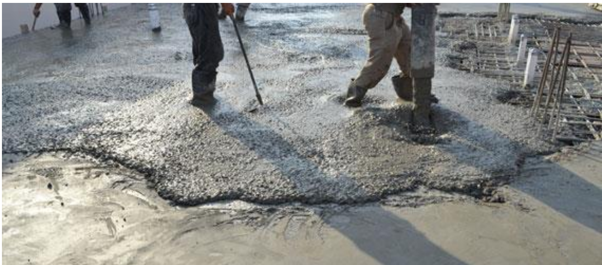
Fig 04: Placing of Concrete
