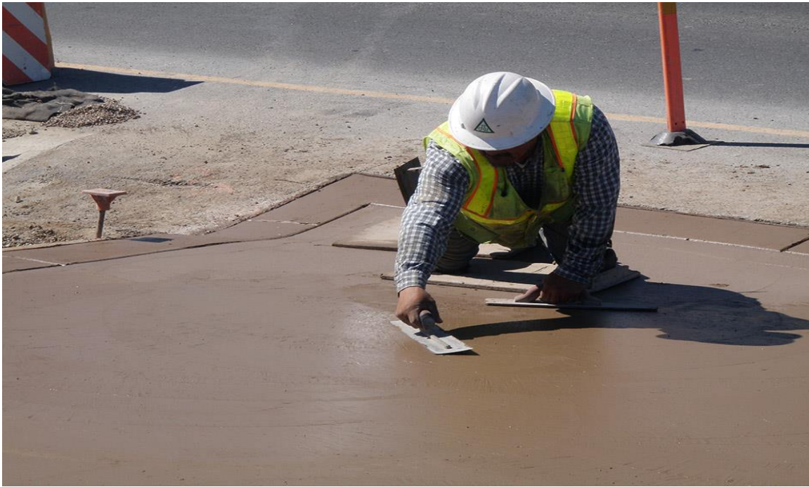
Fig 06: Finishing of Concrete
