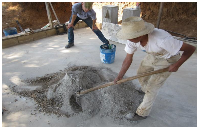
Fig 01: Manual Mixing
