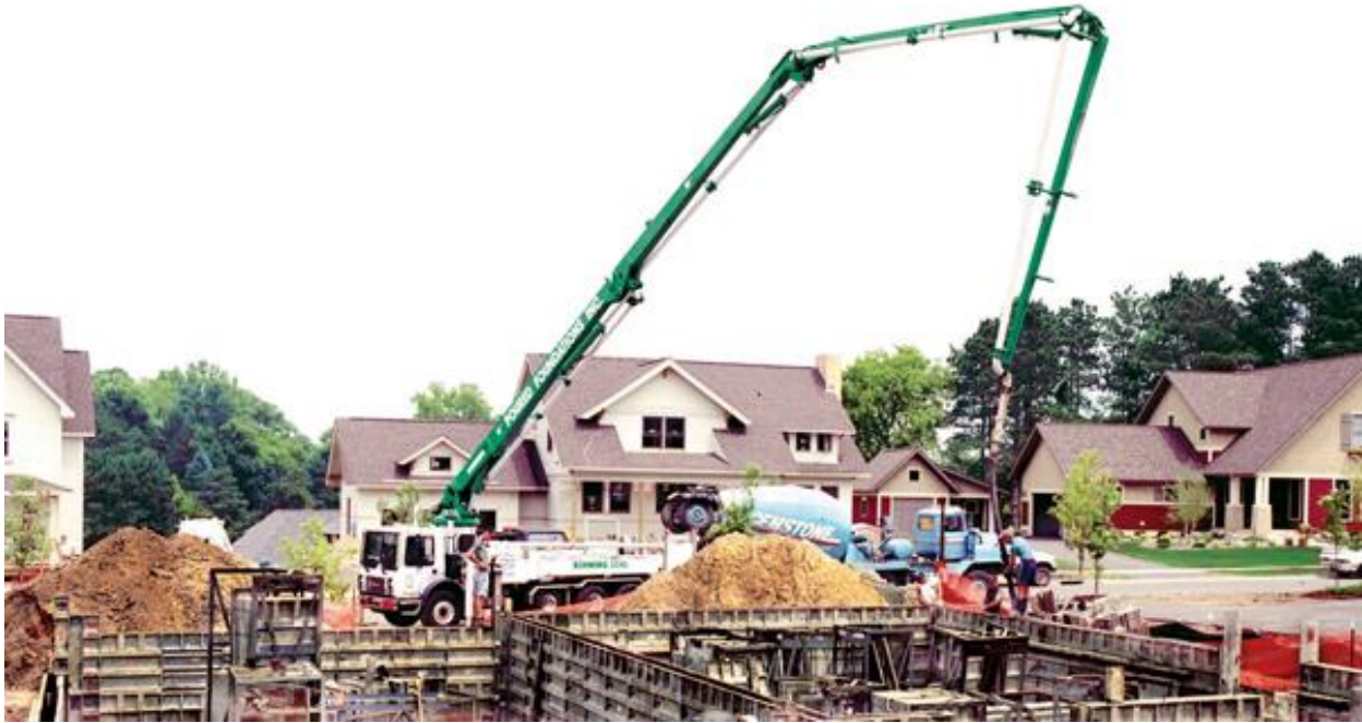
Fig 03: Mechanical Transportation with Pump
