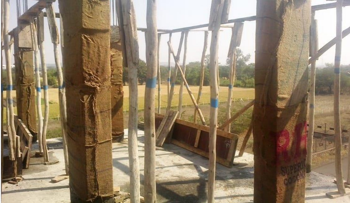
Fig 07: Curing by Wet Jute Bags
