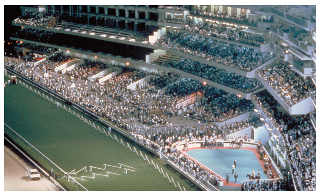
Top Kensington Oval Cricket Stadium, 2007 Cricket World Cup. Architect and Engineer: Arup Associates
