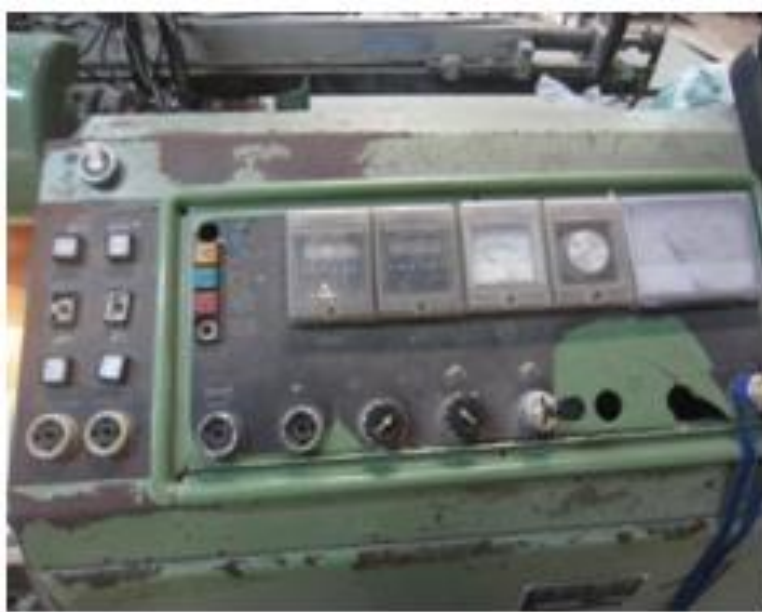
Fig: Control Panel
