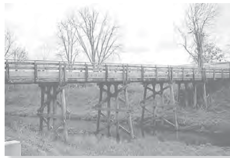
Influence lines for the continuous girder of this trestle were constructed in order to properly design the girder.
