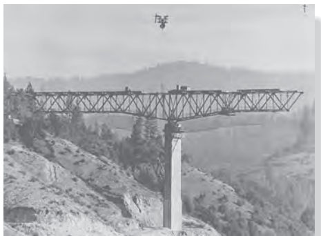
A truss bridge being constructed over Lake Shasta in northern California.
