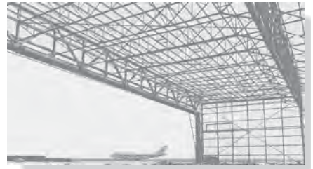
The structural framework of this aircraft hangar is constructed entirely of trusses in order to reduce significantly the weight of the structure. (Courtesy of Bethlehem Steel Corporation)
