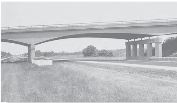
A continuous, reinforced-concrete highway bridge.
