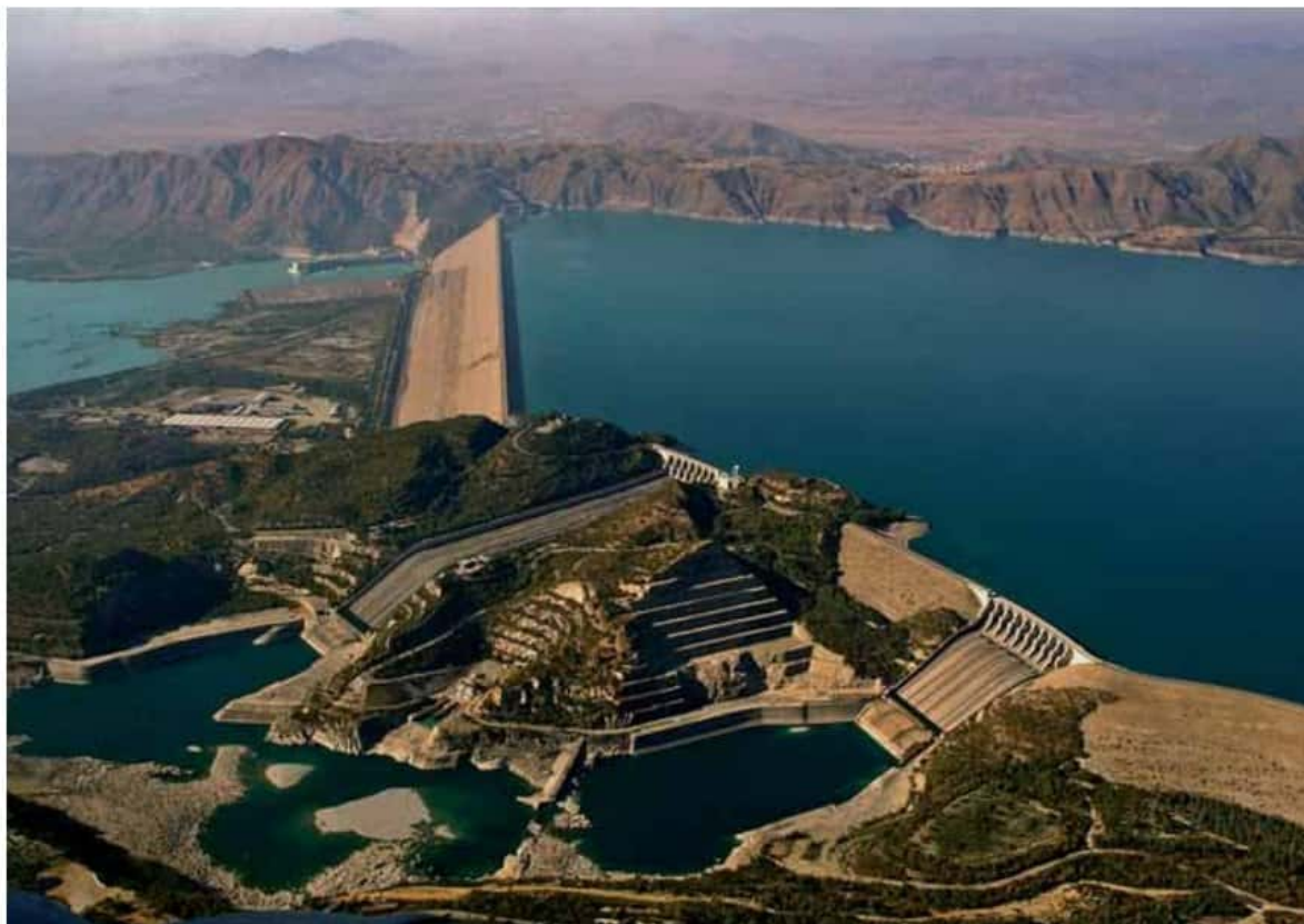
Tarbela Dam, Pakistan's largest, on the River Indus
