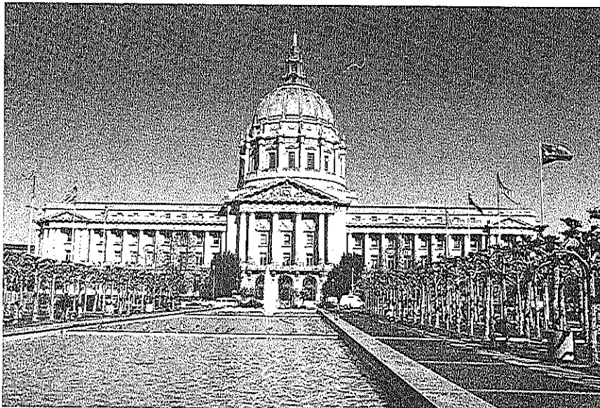
Figure 20.5.1 San Francisco City Hall. (Courtesy of S. Nasseh.)
