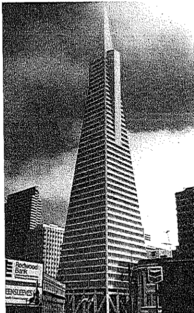
Figure 2.1.2b Transamerica Building, San Francisco, California. The fundamental natural vibration periods of this 60-story steel building, tapered in elevation, are 2.90 sec for north-south vibration and also for east-west vibration. These vibration properties were determined by forced vibration tests. (Courtesy of International Structural Slides.)
