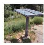
: Tracking solar panel mounts follow the path of the sun during the day to maximize the solar radiation that the solar panels receive. A single axis tracker tracks the sun east to west and a two-axis tracker tracks the daily east to west movement of the sun and the seasonal declination movement of the sun.
