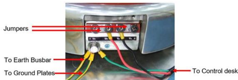
Fig. 1.5 HV Transformer Connections
