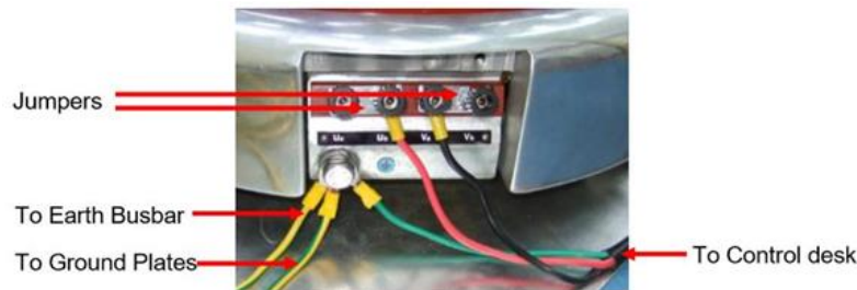
Fig. 1.5 HV Transformer Connections
