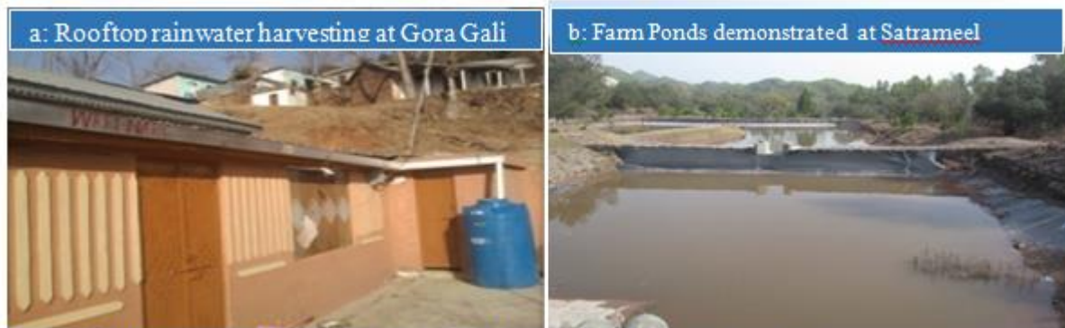
Figure 2: Rainwater Harvesting Systems demonstrated at various sites
