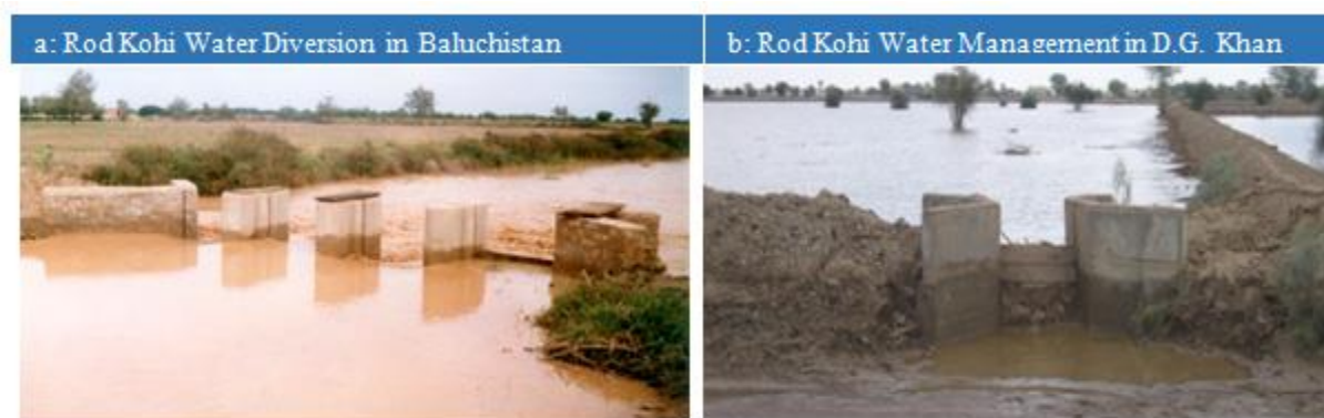
Figure 3: Rod Kohi Management Systems Demonstrated at various sites
