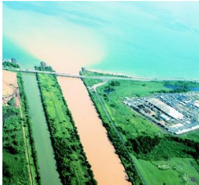
Contrasting side-by-side ditches show the impacts of human-induced sedimentation. The heavily silted ditch carries its load into the coastal waters of San Juan, Puerto Rico.
