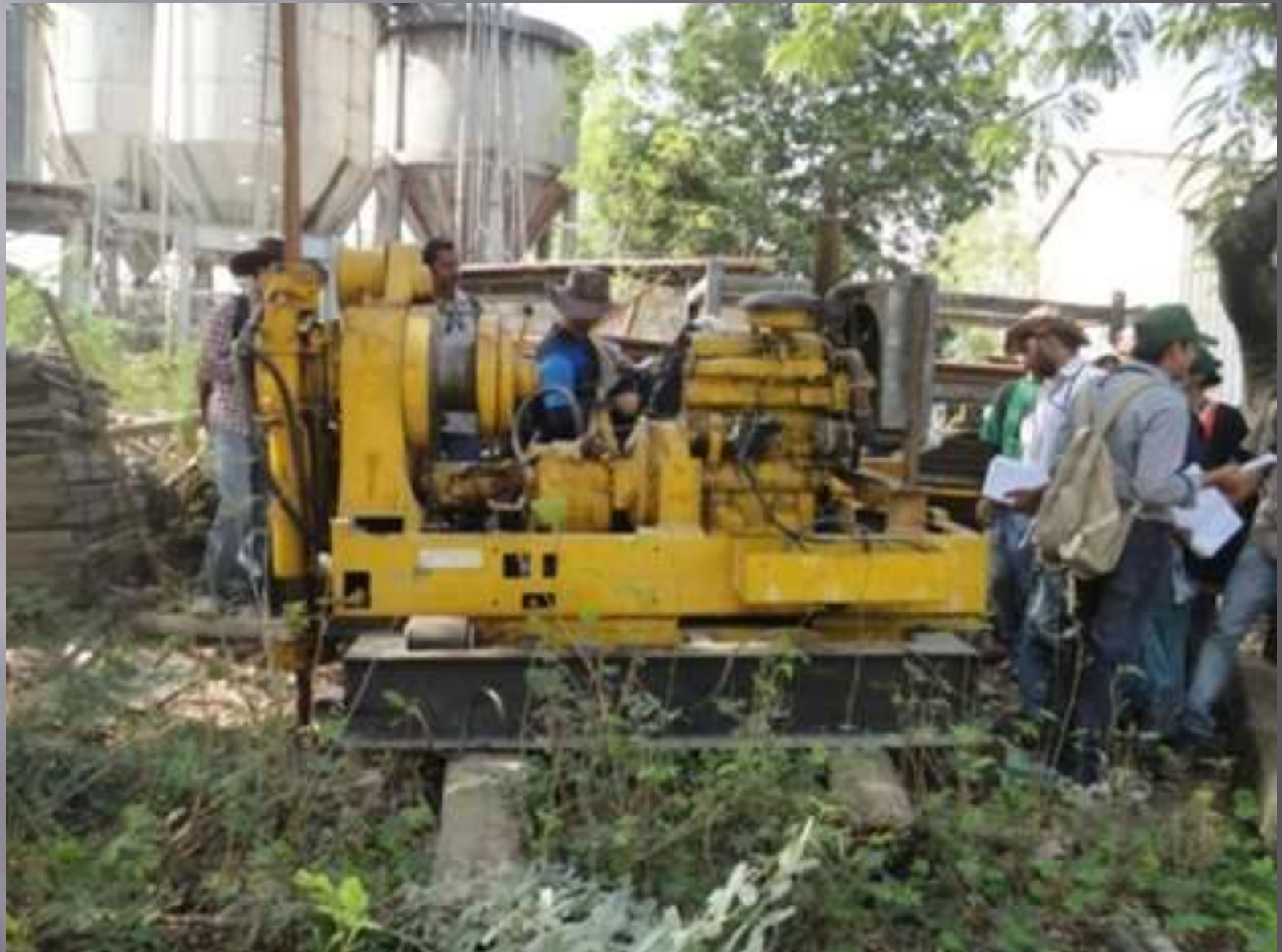
DIAMOND CORE DRILING MACHINE AT HUTTI Model-LT575 drilling
