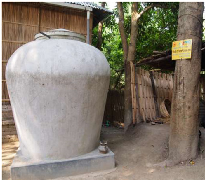
Fig. 9.3 Rainwater harvesting unit
