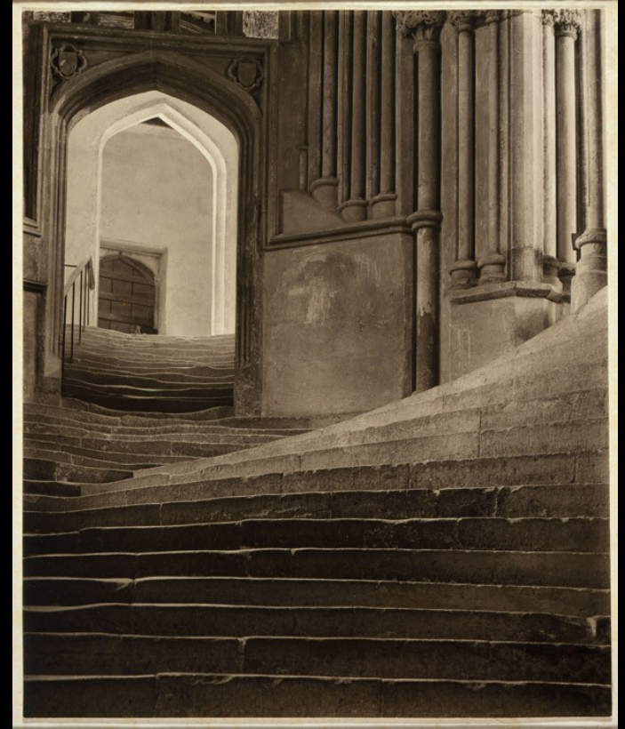
"A sea of steps" stairs to chapter house wells cathedral 1903
