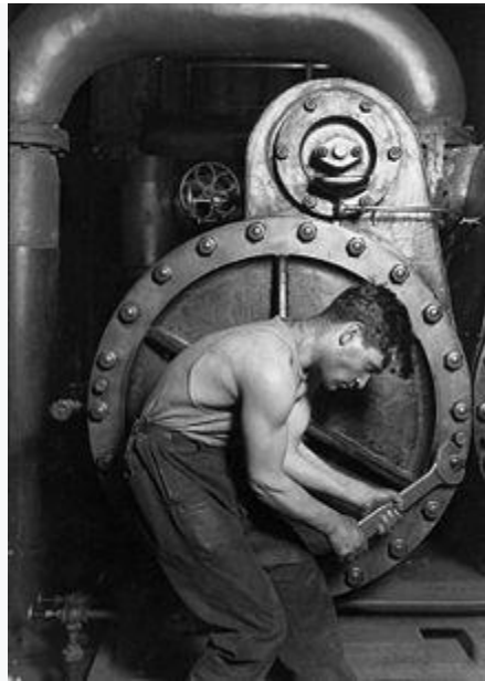
Power house mechanic working on steam pump (1920) by Lewis Hine
