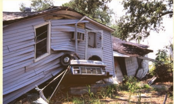
Flood damage left after Hurricane Katrina hit New Orleans.
