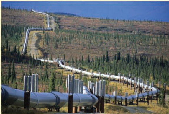
Oil pipeline on refrigerated piles across permafrost, Alaska.
