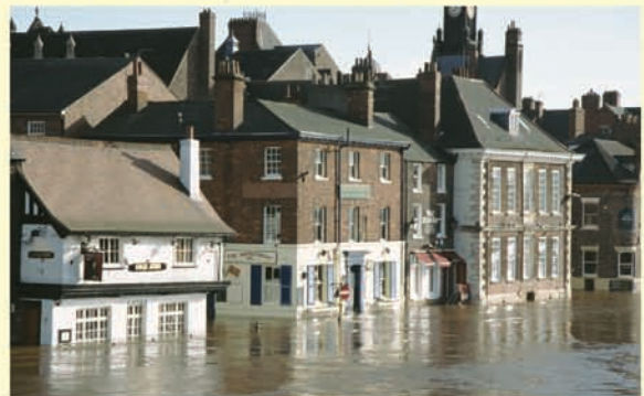
Houses under water on the active floodplain through York.
