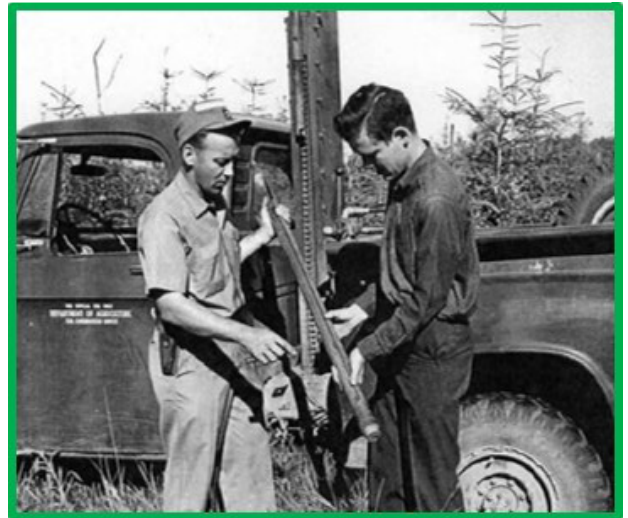
[Figure 1: Albin Martinson and Donald Owens using a truck mounted hydraulic probe]
