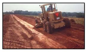
Soil excavated when forming the channel is used to construct the berm
