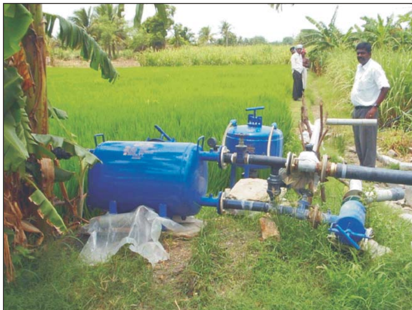
Fig. 15.17 Drip fertigation unit–sugarcane
