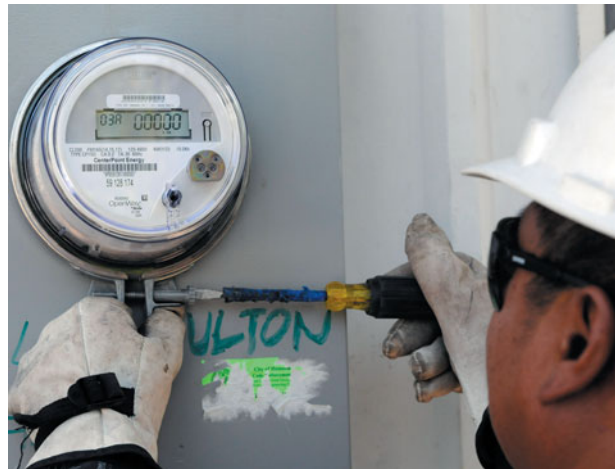
A smart meter being installed
