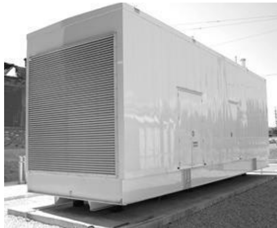
Picture 8: 2 MW diesel generator
