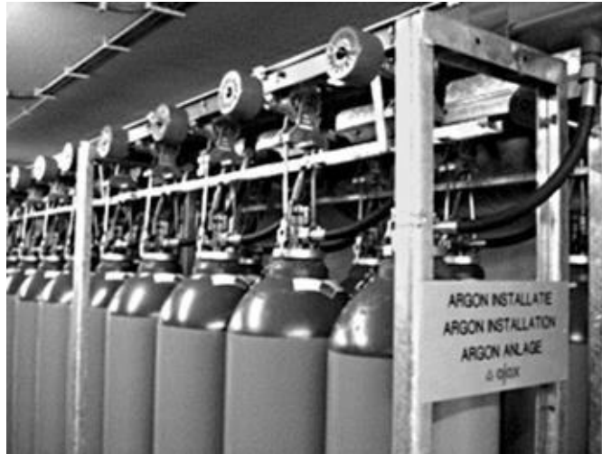
Picture 10: Argon fire suppression system
