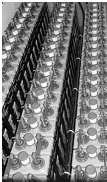
Picture 9: UPS battery array
