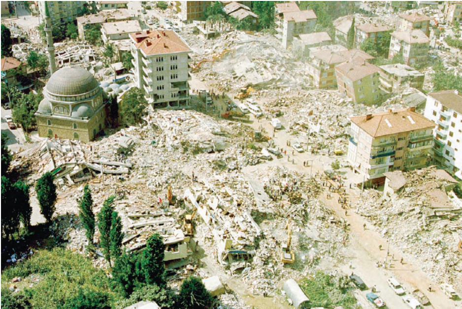
Figure 6.35 Collapse of buildings in Turkey Damage to the town of Golcuk in western Turkey from the M 7.4 earthquake of August 1999. The very old mosque on the left remains standing, whereas many modern buildings collapsed. (Enric Marti/AP/Wide World Photos)
