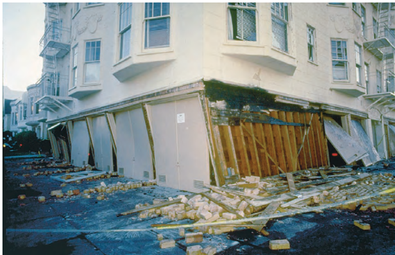
Figure 6.20 Earthquake damage Damage to buildings in the Marina district of San Francisco resulting from the 1989 M 7.1 earthquake. (John K. Nakata/ U.S. Geological Survey)
