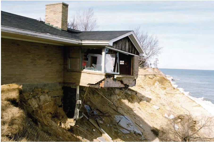
Figure 10.17 Lakes have coastal erosion problems Coastal erosion along the shoreline of Lake Michigan has destroyed this home. (Steve Leonard/Getty Images, Inc.)
