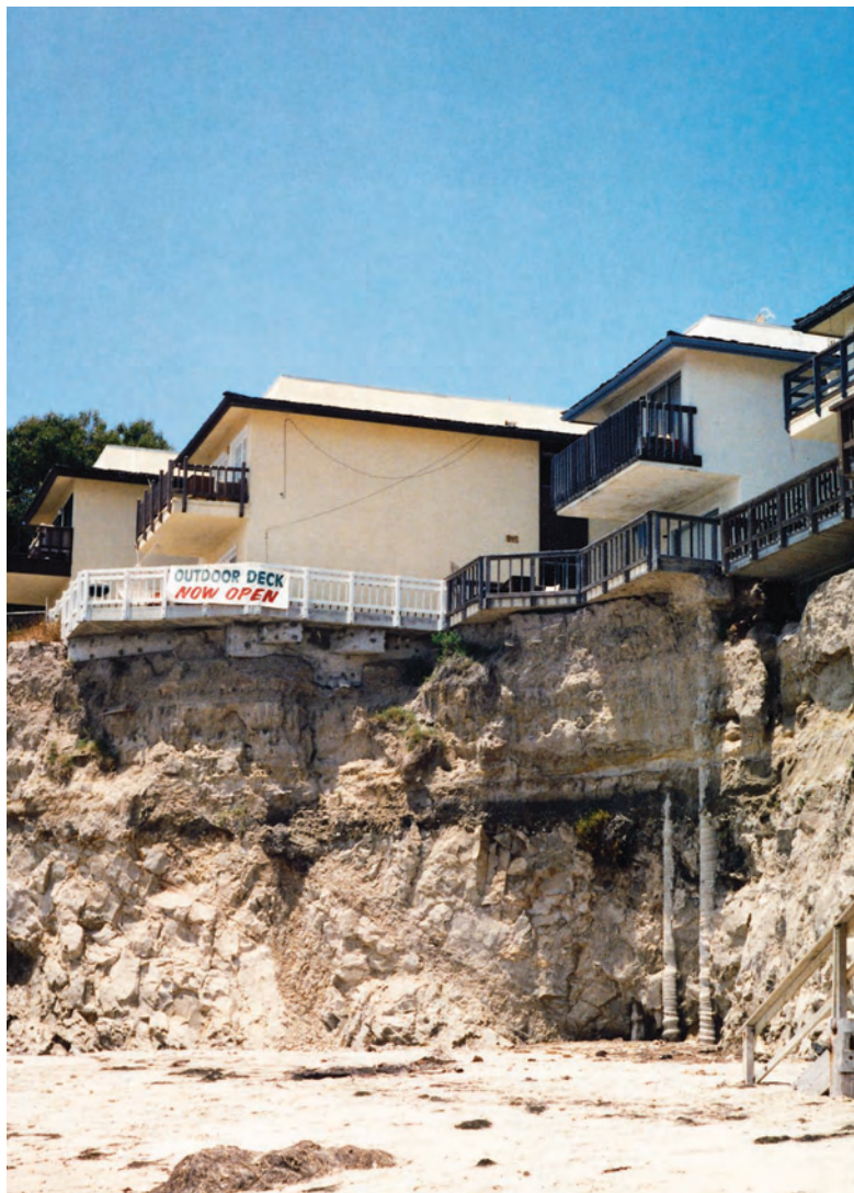
Figure 10.10 Students living on the edge Apartment buildings on the edge of the seacliff in the university community of Isla Vista, California. The sign states that the outdoor deck is now open. Unfortunately, the deck is not particularly safe because it is overhanging the cliff by at least 1 m (3.3 ft). Notice the exposed cement pillars in the seacliff, which were intended to help support the houses. These decks and apartment buildings are in imminent danger of collapsing into the sea. (Edward A. Keller)
