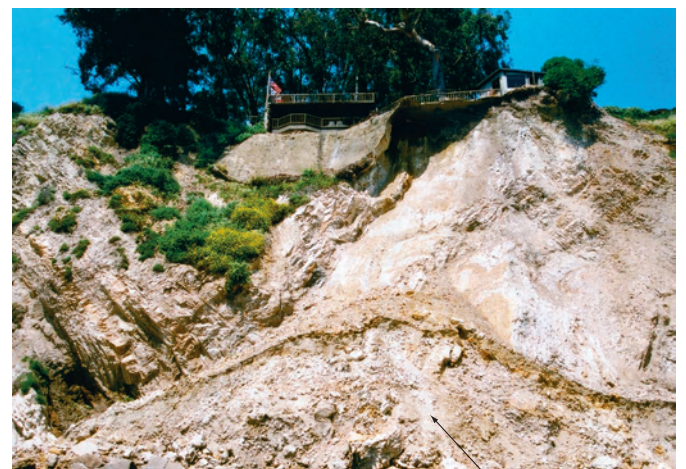
Figure 10.9 Seacliff erosion (a) The pipe in this photograph, from the early 1990s, carries surface runoff from the top of the seacliff down to the beach. Notice that the house at the top of the seacliff has a layer of cement partway down the cliff. The purpose of the cement is to retard erosion. (b) The same location in 2001. Note the landslide that has occurred, removing some of the cement and rock of the seacliff. (Edward A. Keller)
