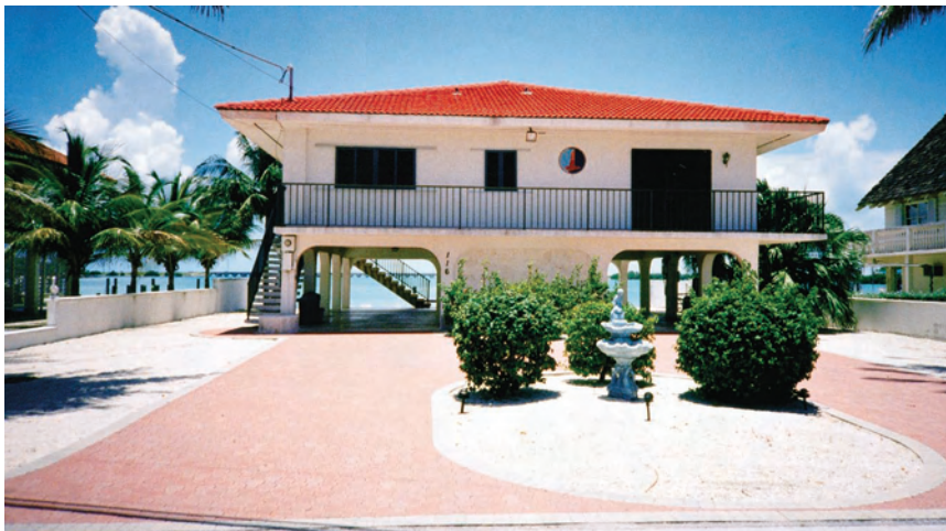
Figure 10.24 Hurricane resistant house Home in the Florida Keys, constructed with strong blocks to withstand hurricane force wind and space below to allow the flow of a storm surge beneath the building. (Edward A. Keller)
